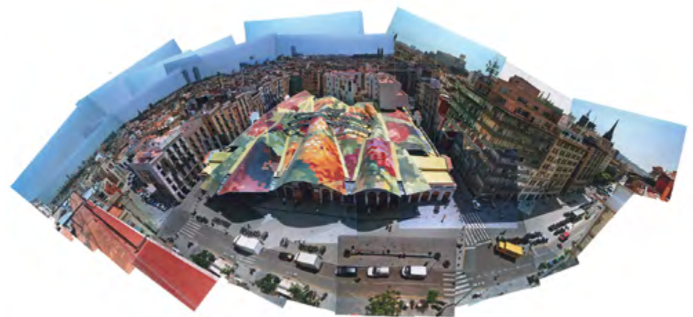
THE ROOF AFTER THE RENOVATION
